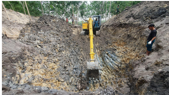
Figure 8: A mechanical excavator removing ex-situ spoil down to undisturbed substratum within an historic bomb crater at the Balmoral search area. Image HTH
